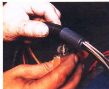
15. The heat of the flame shrank the shrink tube around the convoluted tubing, which makes for a nice wire loom transition.
