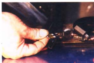
17. The two 30-amp fuses were installed into the fuse holders.
